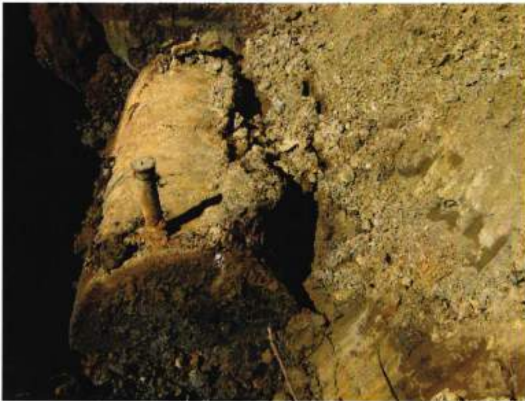
Image 4. 2 K UST – UST in ground, awaiting to be removed.
