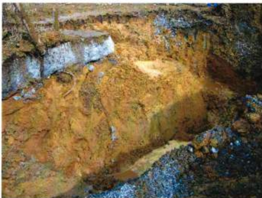
Image 1. 10 K UST- UST in ground with concrete on top.
