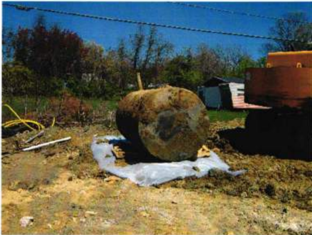
Image 5. 2 K UST – UST removed from the ground , awaiting final disposal.
