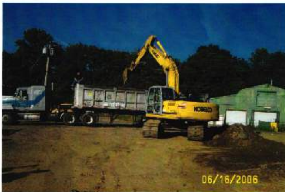
Image 7. Disposal of "contaminated" soil to disposal facility.
