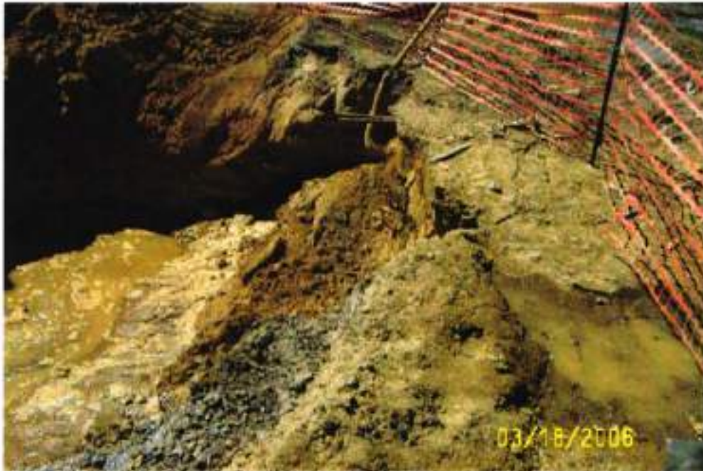
Image 3. 10 K UST – Post Excavation hole.
