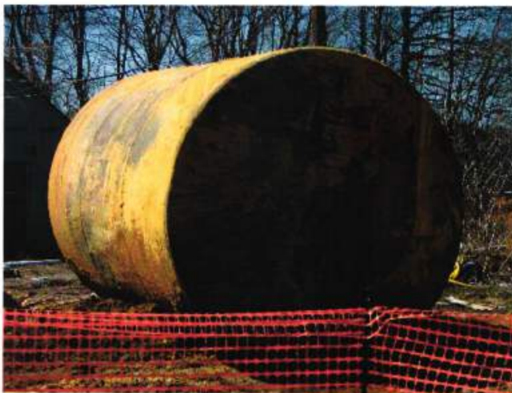
Image 2. 10 K UST – Tank sitting on ground awaiting final disposal.
